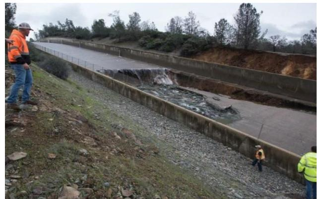
Fig. 2: spillway in operation, damaged spillway
