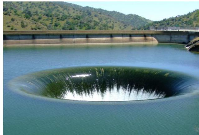
Fig. 1: stepped spillway with chute blocks, morning glory spillway
